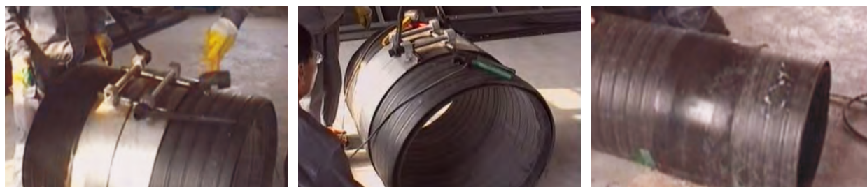
4. use clamp and buckle fix the welding piece
