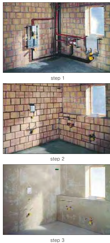
© Installation plan for the lightweight brick wall structure
