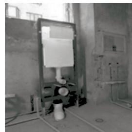
2. Installation of water tank and support
