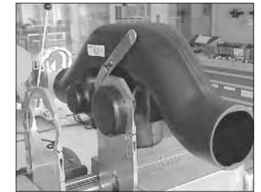
2、 Install the fitting into the welding machine
