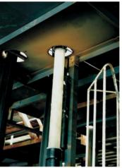
Kingbull's patented Siphionic roof outlet could help to achieve siphonic effects with less rainwater on the roof, therefore protecting roof from overloading. It is completed with simple and stylish appearance and a unique corrosion resistance treatment to improve surface corrosion resistance
