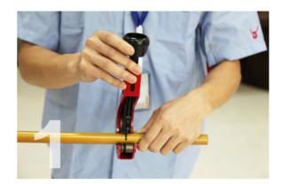
Cut off Kingbull pipe vertically with pipe cutter, make sure that the cross section must be vertical to the axis.
