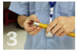
Choose the right size fitting, push the inserts into the pipe up to the baffle ring until the pipe is visible through the inspection windows, and take care not to damage the o-ring.
